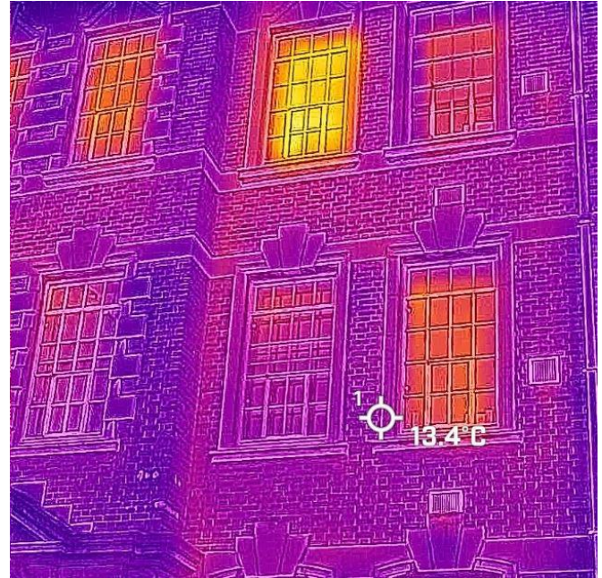
Thermal Imaging Survey conducted on the building prior to the Secondary Glazing project
