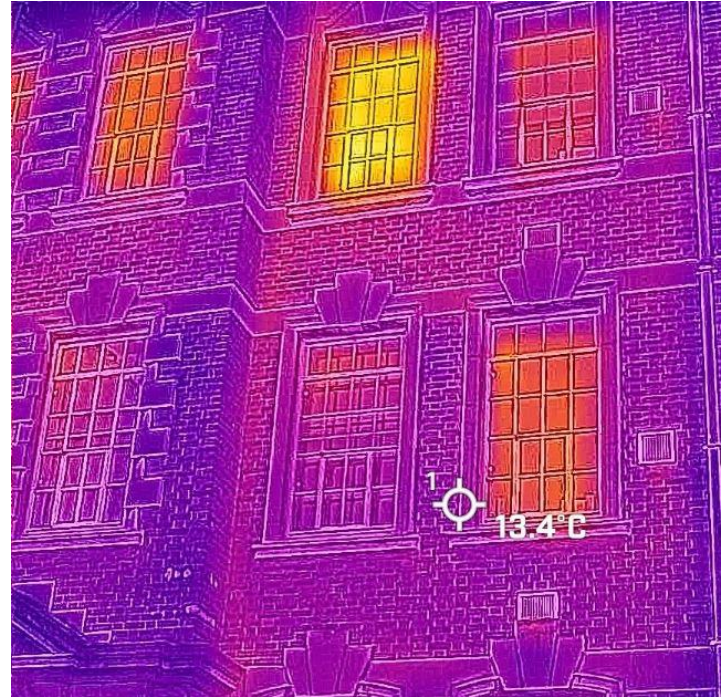
Thermal Imaging Survey conducted on the building prior to the Secondary Glazing project
